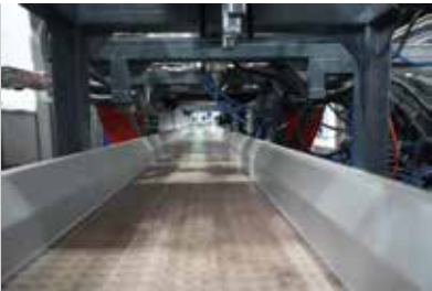
HS-Waste Material Recycling System
